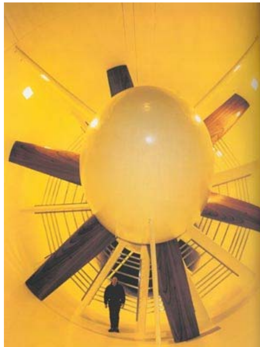
Figure 4-7 : Le fan principal
